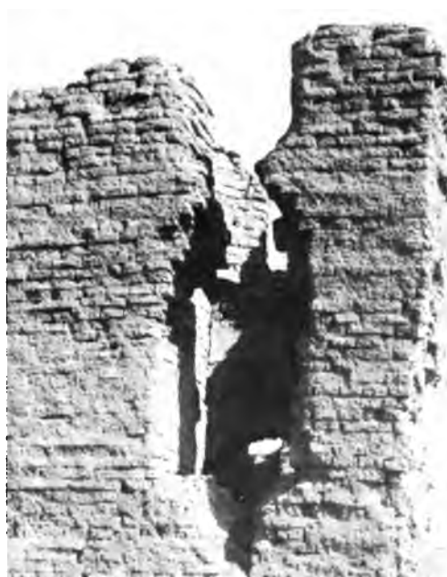
(d) The domed church, southeast. Cupola from outside.
